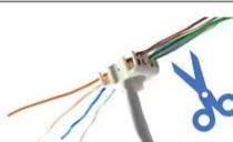
Insert the cable into the termination cap, fan out the conductors in the proper connection slots accordingly colour code.
